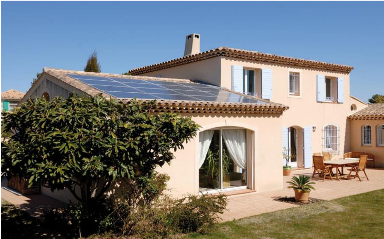
Figure 22 – Example of an excellent installation with PV modules integrated in the rooftop
