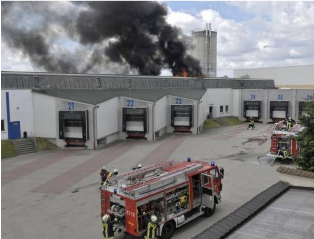
Figure 5 – Example of fire originated in the PV array on a rooftop
